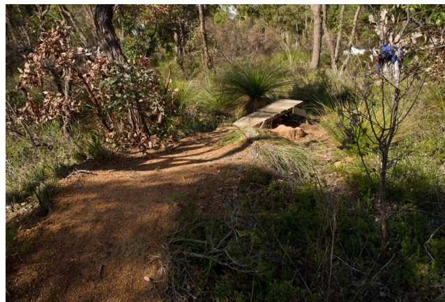
A bicycle jump ramp constructed at site four
