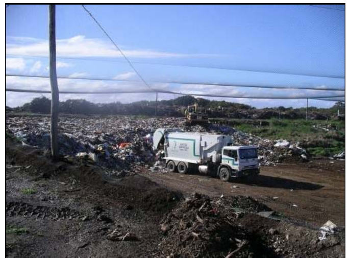
Figure 2 Netting over an active cell at Ballina Landfill (image from Patrick 2006, pg 41).
