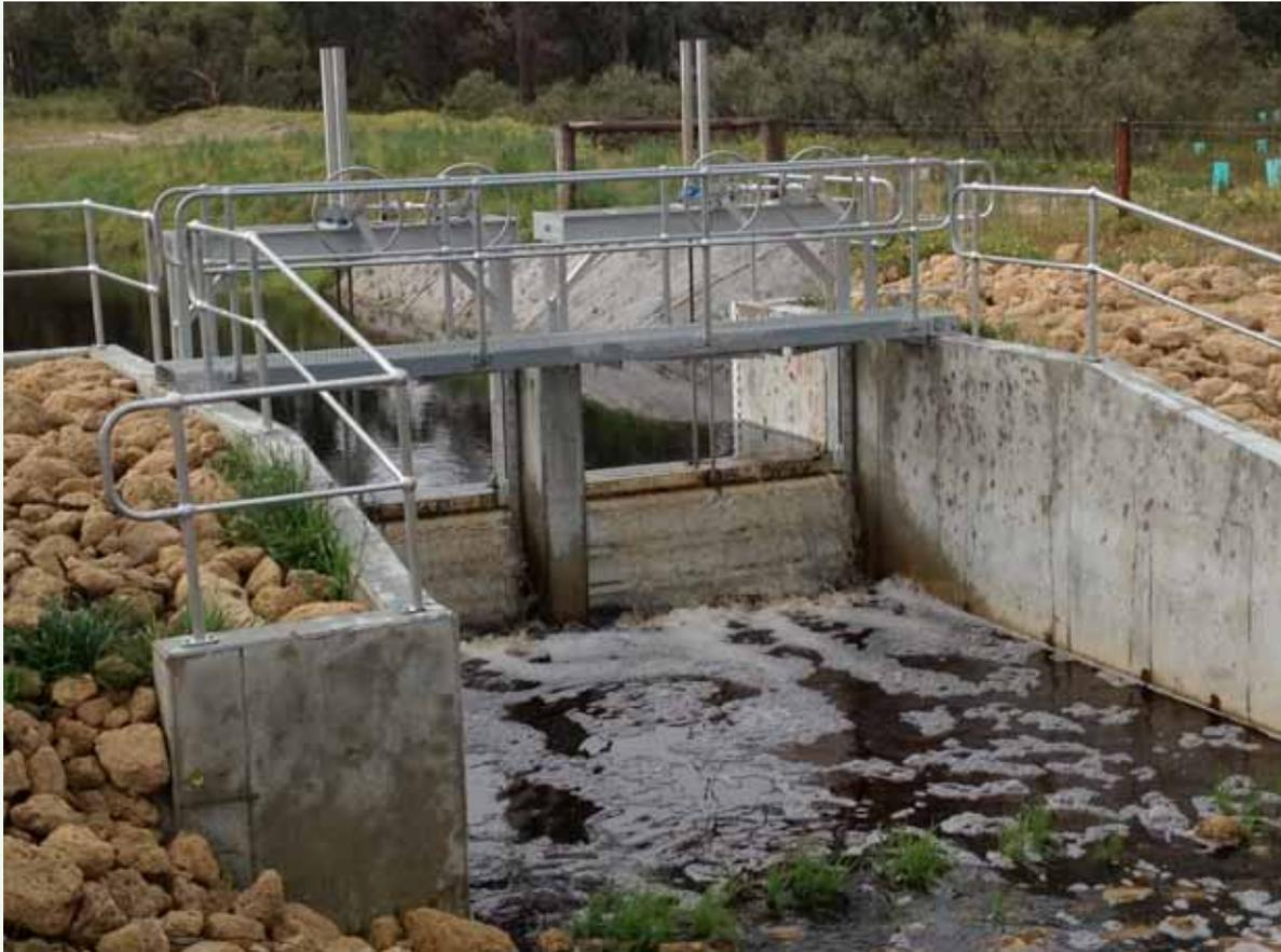
Figure 9. The adjustable height weir, receiving flows diverted from the Mealup Main Drain. Photo – H Bucktin/DEC.
