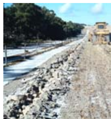
Figure 15. An open rip line is an unsuitable surface for effective herbicide weed control. Image shows a dozer implementing a single rip line. Also note the subsoil boulders in the centre of the rip line are now mixed with the topsoil. This is a result, in part, of excessive ripping depth.
